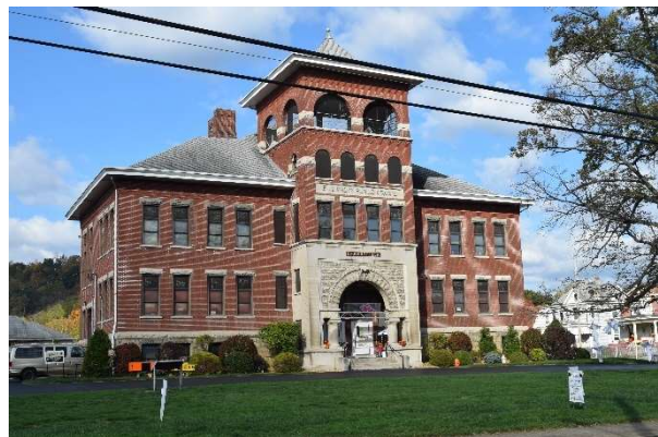
Fig. 24. 144 Kruger Street, former Kruger Street School now used as a museum (OH-0001-0305), 2020.
