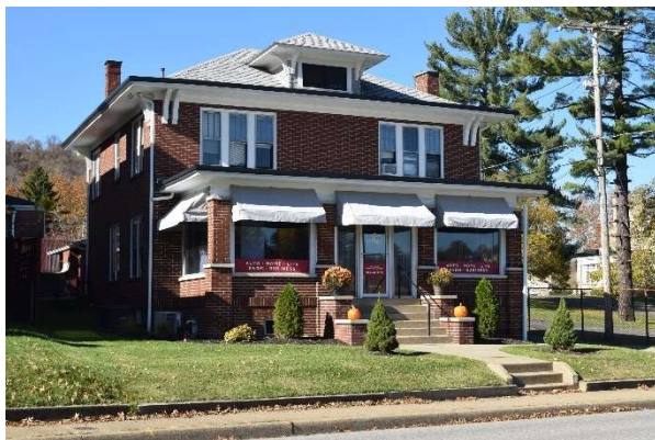
Fig. 23. 1 Kruger Street, former residence now used as office space (OH-0001-0338), 2020.
