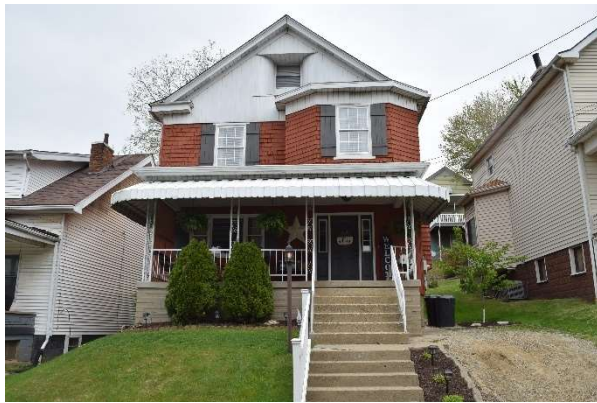
Fig. 38. 119 Cracraft Avenue (OH-1288), 2020.
