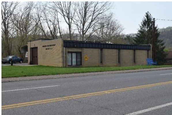
Fig. 26. Wheeling Fire Engine Co. 11, 131 East Bethlehem Boulevard (OH-1213), 2020.
