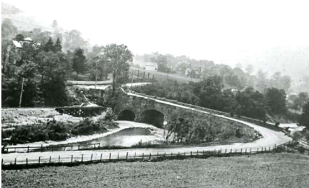
Fig. 5. 'S' Bridge over Little Wheeling Creek, looking west, 1886 (West Virginia & Regional History Center).
