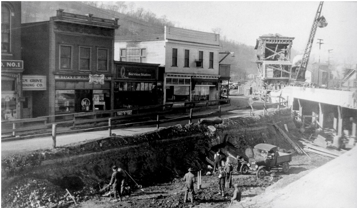
Fig. 14. Excavation of National Road to accommodate train trestle, 1920s. (Weelunk)
