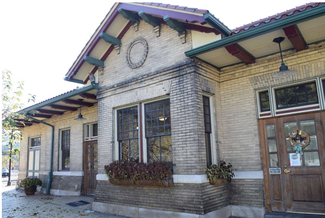
Fig. 46. Former B&O train depot, 2167 National Road (OH-0001-0013), 2020.
