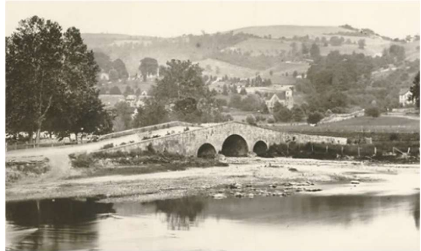
Fig. 6. Stone Bridge on National Road looking southeast, 1888. (Ohio County Public Library)
